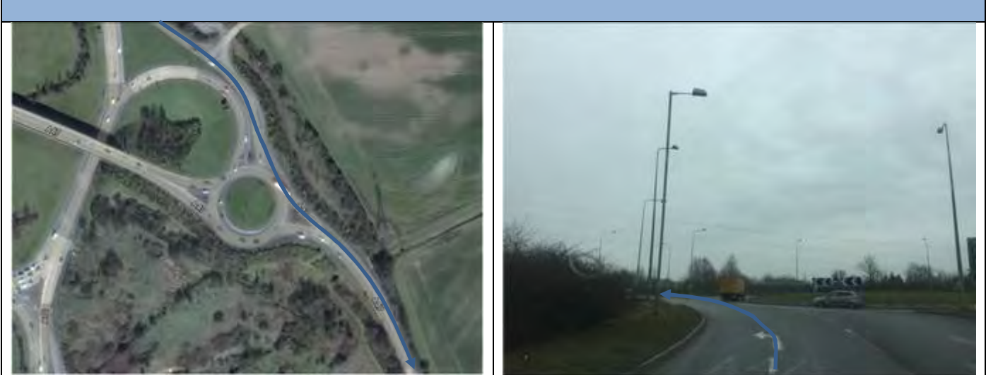
8.7.3.1. – Aerial View of Location 8.7.3.2. – View of entrance to roundabout
