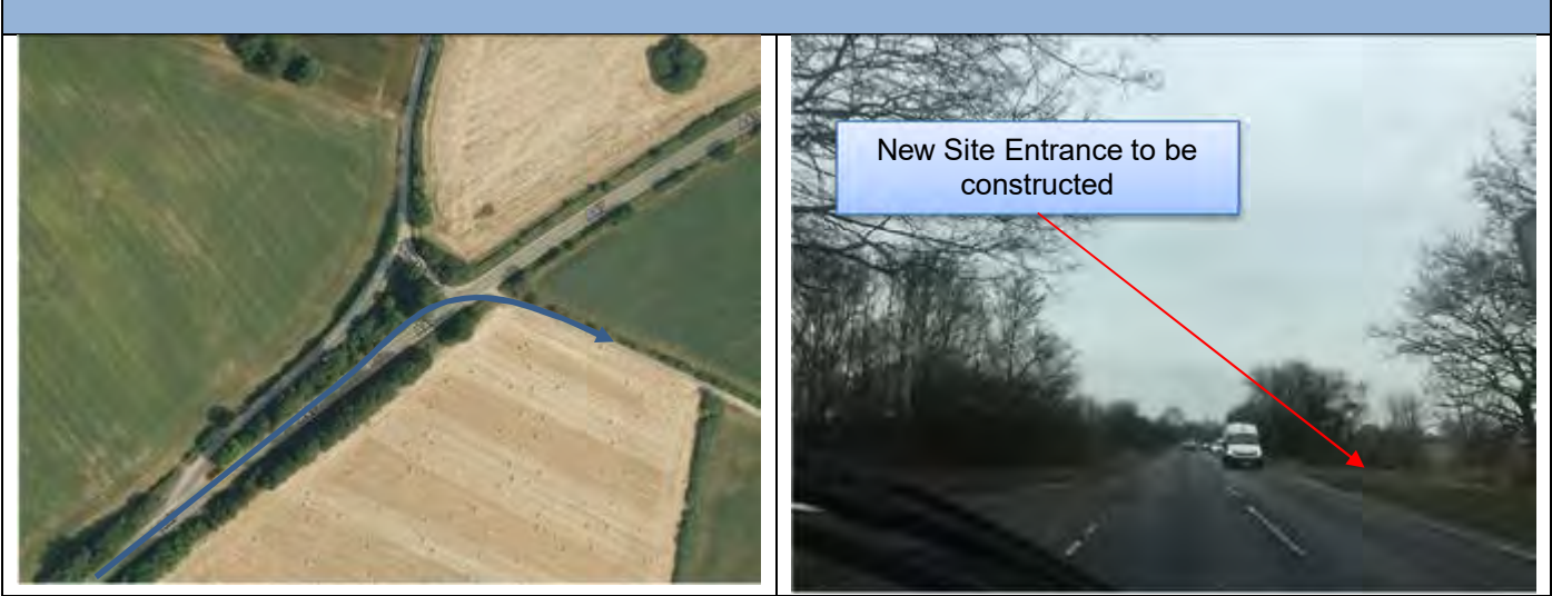
8.8.5.1. – Aerial View of Location 8.8.5.2. – View of entrance to roundabout 8.8.5.3. – View on roundabout
