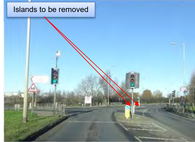
8.4.6.3. – View on junction
