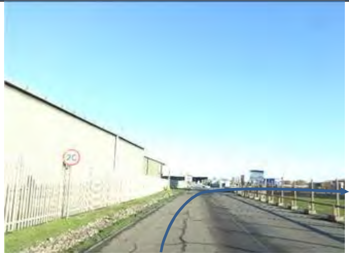
8.4.2.2. – View prior to bend
